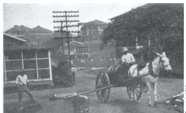
Figure 5. Laborers controlling mosquito larvae by applying crude oil to roadside drainage ditches in the Panama Canal Zone using a pipe apparatus, circa 1912
