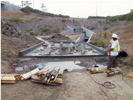
Fig. 7.4 An extended detention basin retrofit.
