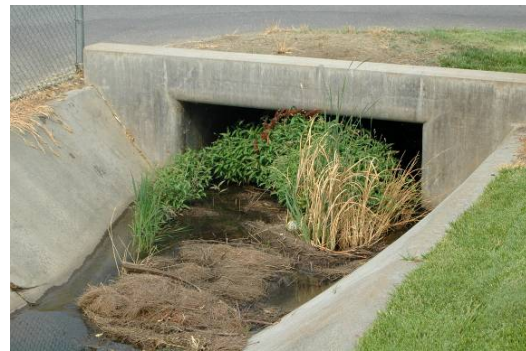
Fig. 7.3 A poorly maintained culvert under a public street
